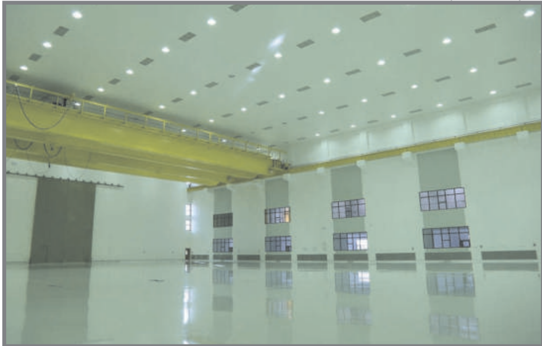
Metal false ceiling & Epoxy PU Painting
