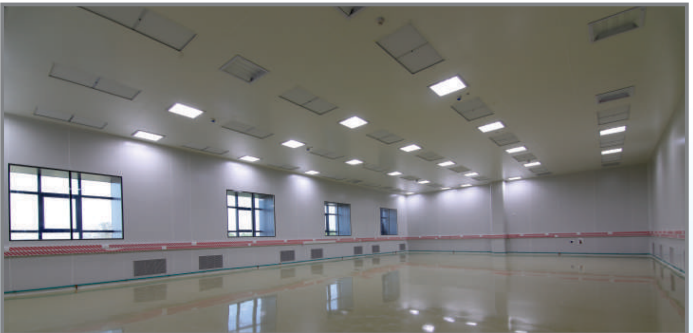
Clean room of 1,00,000 class with Antistatic Flooring at Vendor Complex, ISRO
