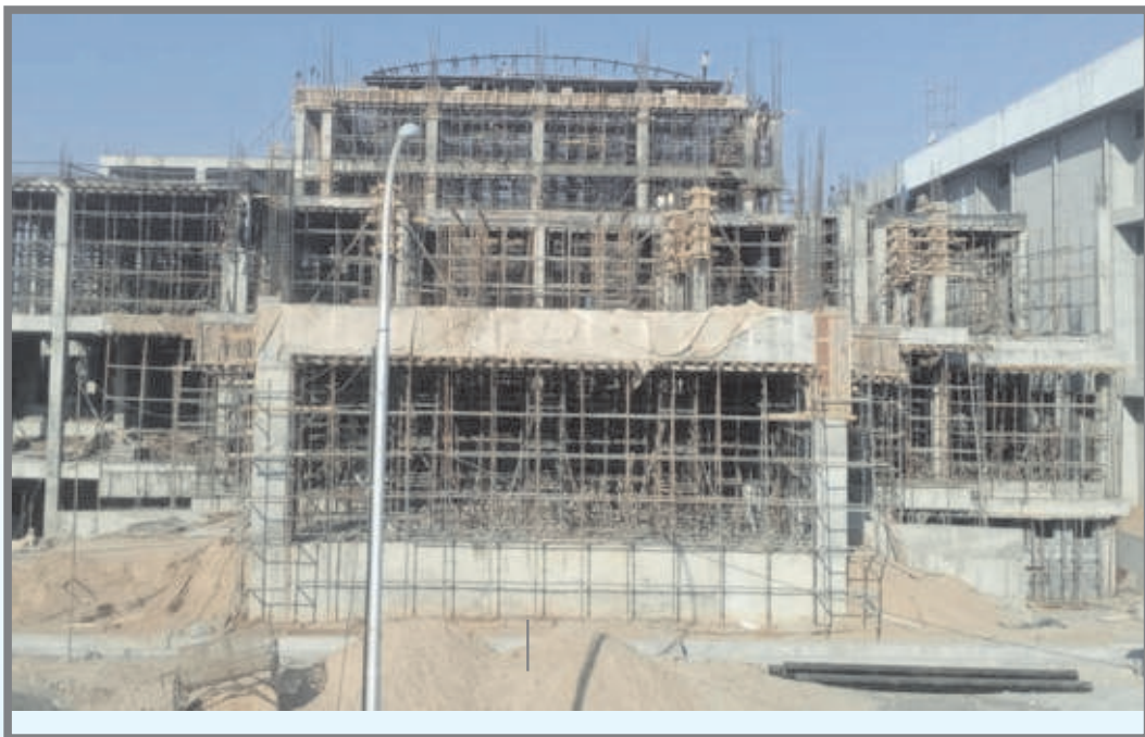
Highbay slab staging at 24 Mtr. Height
