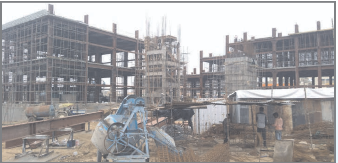
Mezzanine Floor work at Vendor Complex, ISRO
