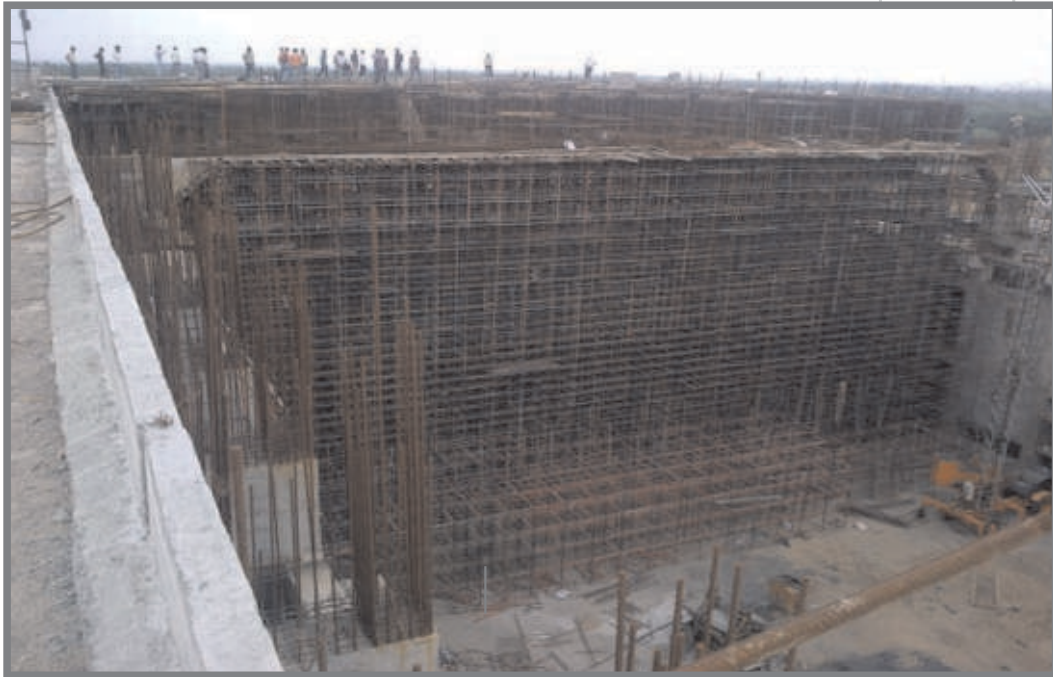
Highbay slab scaffolding @ 23 Mtr. Height
