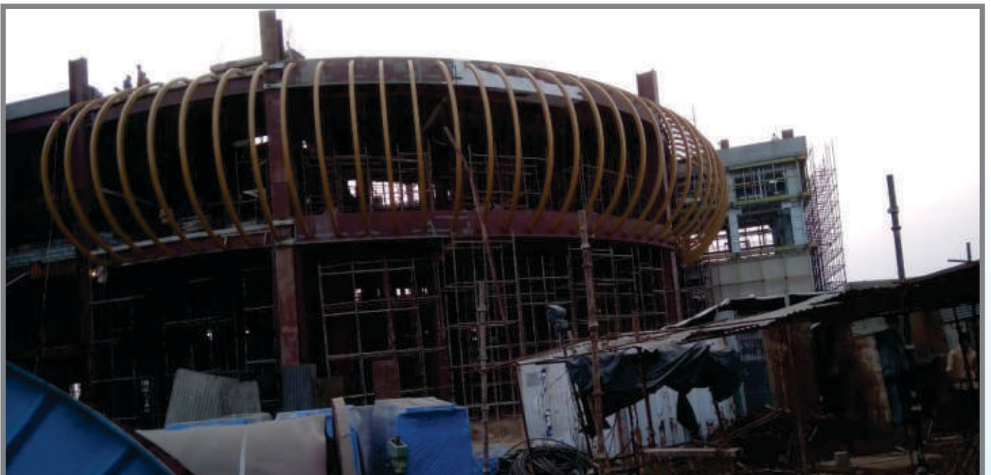
3 Dimension curved glass structure at Vendor Complex, ISRO
