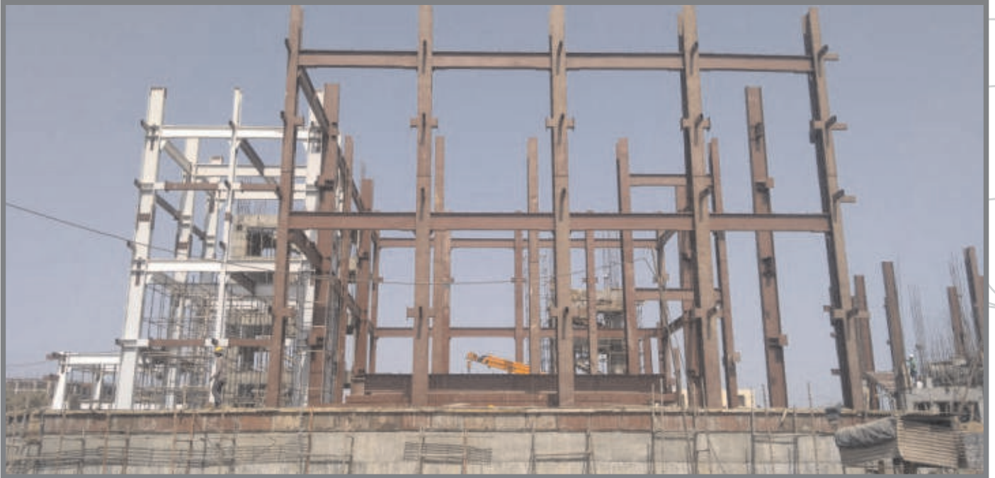
Heavy Steel Structure work at Vendor Complex, ISRO
