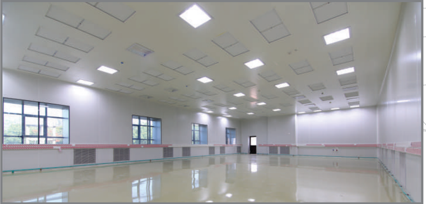
Clean room of 10,000 class with Antistatic Flooring at Vendor Complex, ISRO
