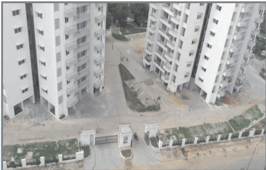
Infrastructure work at Godrej Properties Ltd.
