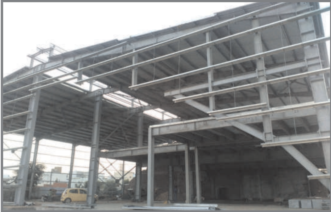
PEB work for Indoor Sports Complex (SAG)
